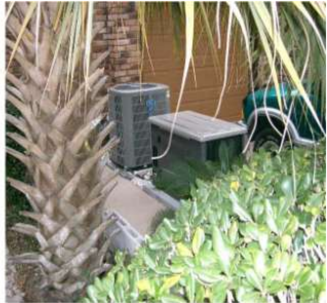
Generator (Interior Front) Unit 208
